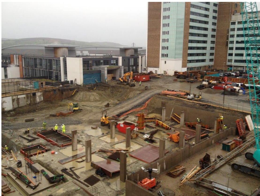
Construction underway at the Radiotherapy Centre at Altnagelvin Hospital, Derry.
